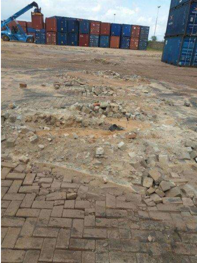
Example of tire damage
