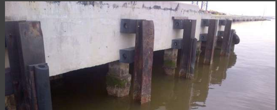
Waterline Fenders and Piles
