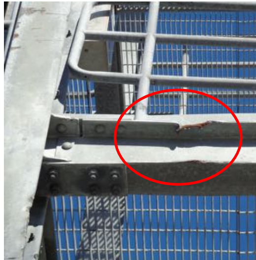
Damaged beam flanges
