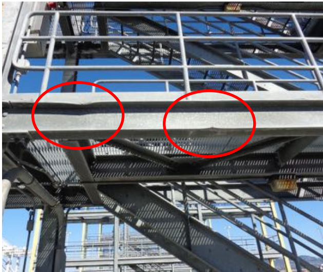
Bent beam flange
