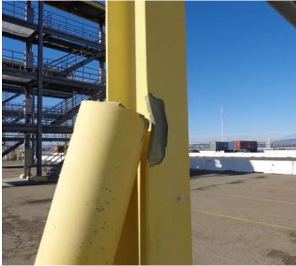
Mechanical damage to column
