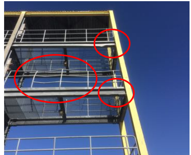
Bent beam flanges and guardrails
