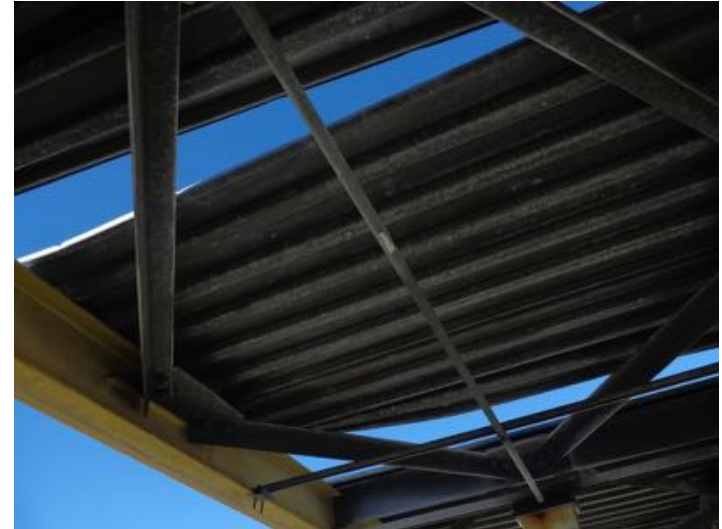
Gaps in roof deck
