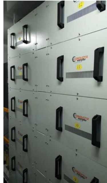
Battery modules inside the housing
