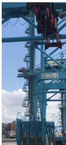
Fig. 5: test 1-2, 30t 2-Corner South
